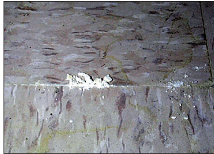
The effects of elevated pH levels can be seen in these examples of re-emulsified adhesive, soluble salts, and blistered floor coating.
