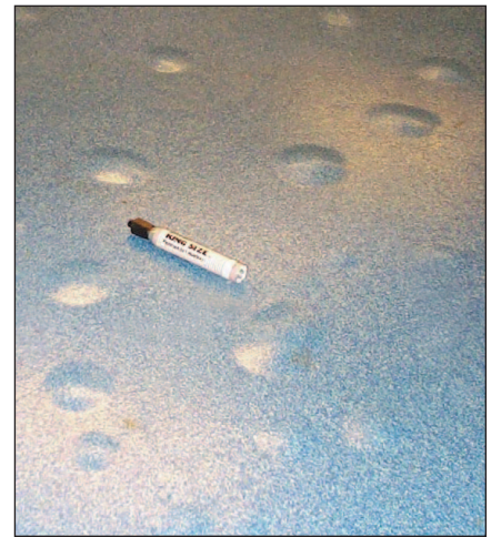
The effects of elevated pH levels can be seen in these examples of re-emulsified adhesive, soluble salts, and blistered floor coating.
