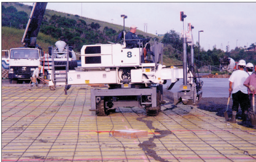
A thicker vapor barrier is required where there will be equipment traffic or with angular base materials. Note the example of torn 6-mil poly.
